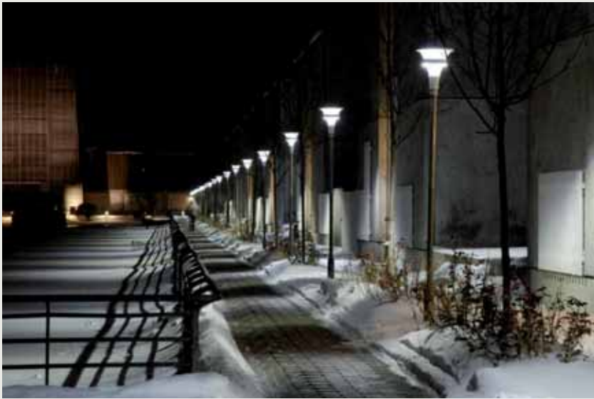
Figure 7: Albertslund street lighting (© City of Albertslund)
