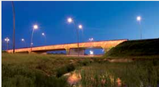
Figure 2: Bridge Lighting in Eindhoven 22 (© City of Eindhoven)
