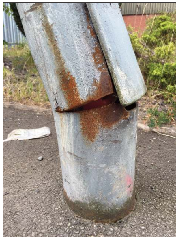
Picture A12.28: Crack from edge of door opening
