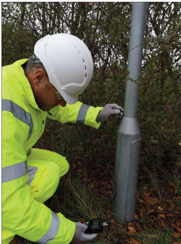
Picture A1.4: Ultrasonic testing
