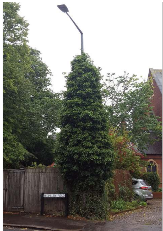
Picture A12.38: Significant ivy growth on concrete column
