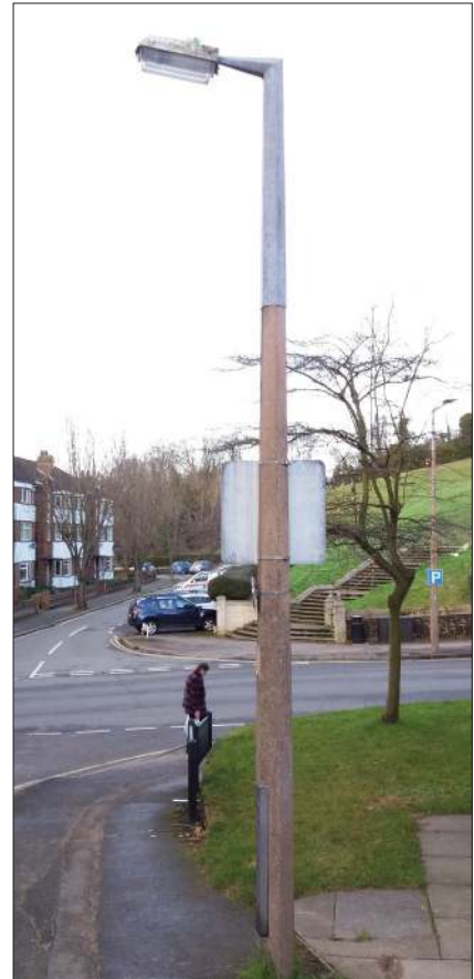
Picture A12.16: Sleeved 5m concrete column
