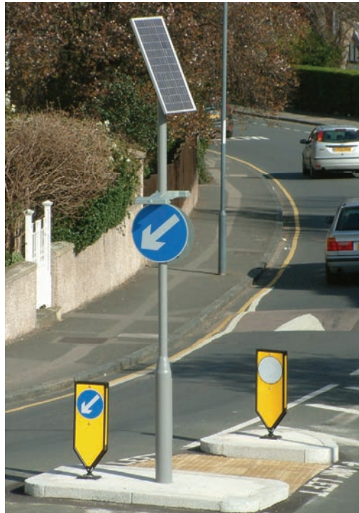
Figure 21 – A traffic island installed without requiring mains electricity cabling and connection
