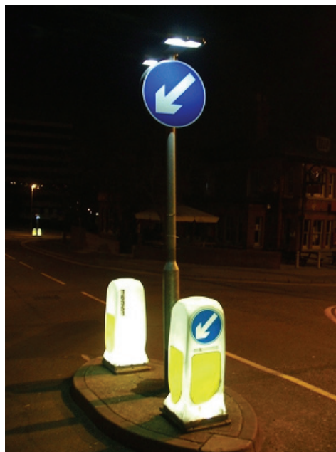
Figure 16 – Bollards used in combination with a D610 ‘keep left’ arrow to form a traffic island
